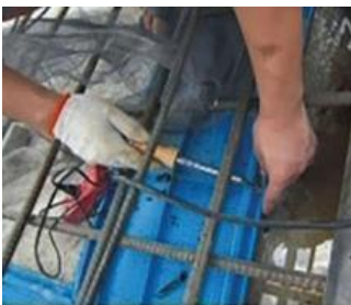
INSTALLATION OF EXTERNAL WATERSTOP
