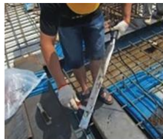
INSTALLATION OF EXTERNAL WATERSTOP
