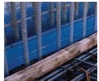
INSTALLATION OF BUILT-IN WATERSTOP
