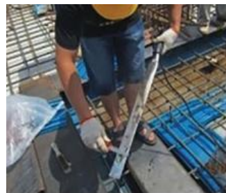
INSTALLATION OF EXTERNAL WATERSTOP
