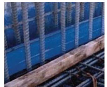
INSTALLATION OF BUILT-IN WATERSTOP
